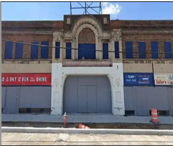
In 2015–2016, the former Moreland Theatre site and adjacent to E119th Street and Buckeye Road were abandoned and deteriorating. Essentially, the dilapidated buildings were covered with an ugly blue-gray paint as if alerting developers that the neighborhood was ripe for urban removal projects. LAND Studios was responsible for this project.How much money was spent on “art”that could have been spent fixing the properties? Then more murals were painted. Then the trash cans were painted. Later, Cleveland Neighborhood Progress used funds, an undisclosed amount, to paint the trash can, twice,along Buckeye Road. Ten years later, the area looks like a war zone. while millions of development dollars cannot be accounted for.
